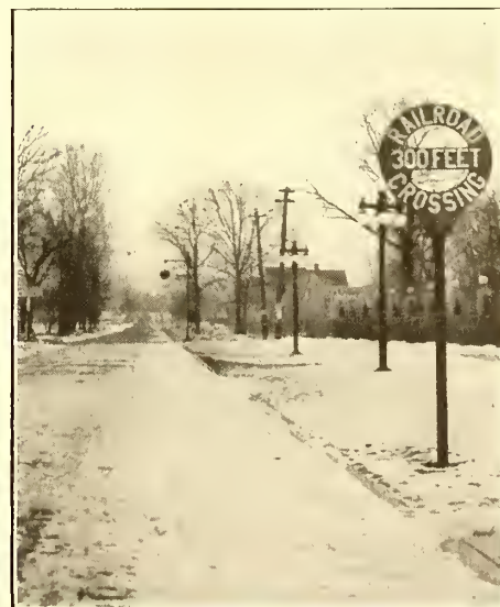
NORTH SHORE GRADE-CROSSING PROTECTION—AUTOMATIC WIG-WAG SIGNAL AND SIGN INSTALLED AT CROSSING AND WARNING SIGNAL INSTALLED 300 FT. AWAY
